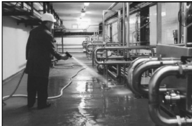
Manual cleaning using trigger-action guns on hoses
