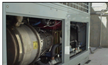
STM Stirling Engine Generator (Beta version), 25 kW Case Open
