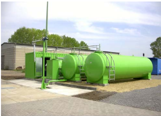
Biodiesel plant in Germany (900 t/a capacity)
